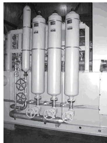
LOSAs designed per ASME Sec. VIII, Div. 1 and National Board Registered
