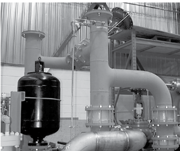
LOSAs designed per ASME Sec. VIII, Div. 1 and National Board Registered
